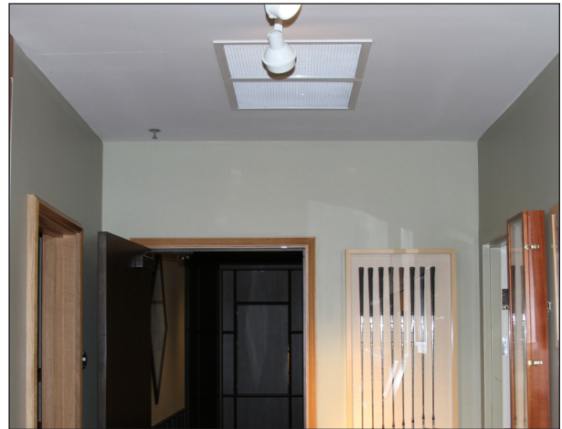
45F grilles installed in the ceiling of a gift shop
